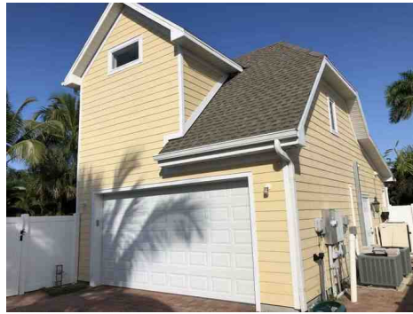
Rear Garage Entry
